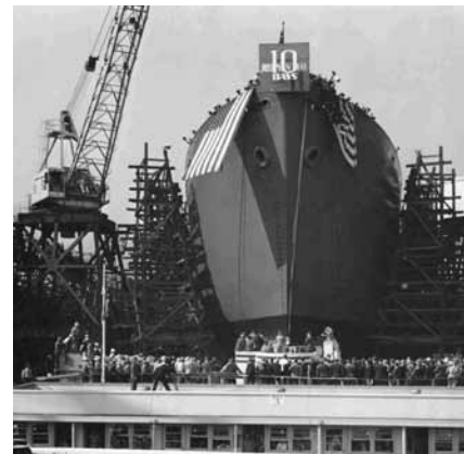
Figure 40. The Kaiser Shipyard in Richmond, California could build and launch a prefabricated cargo ship in about four days. Image courtesy of Library of Congress.
