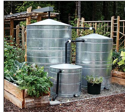
Above-Ground Cisterns Source: Sunset Publishing Corporation
