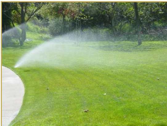
Rotor sprinklers watering lawn. Low precipitation rate.
