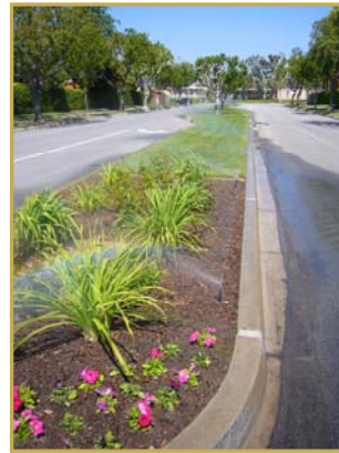
This is an example of poor design. This irrigation station is watering three different plant types that have varying water needs, including lawn, shrubs, and annual flowers.
